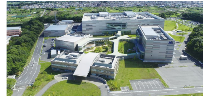
Full view of the H.U. Bioness Complex
