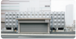
Water storage: Laboratory Building water tank
