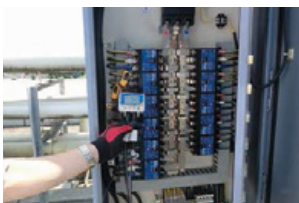
Installing measuring equipment
