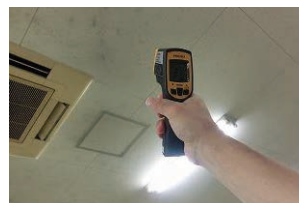
Checking thermal insulation of warehouse ceiling
