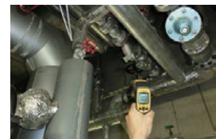
Checking insulation capacity of steam pipe valves
