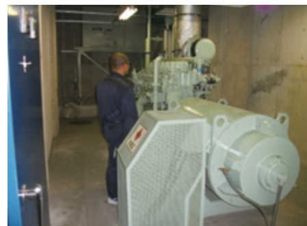
500 kW emergency power generator in the basement of A-bldg.
