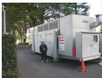
1000kW Temporary emergency power generator
