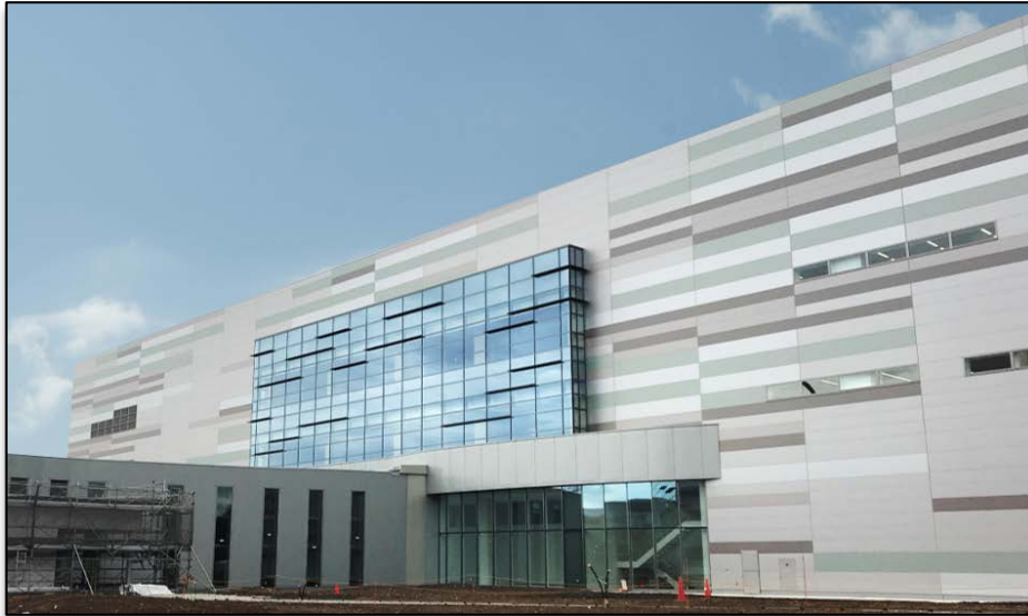
New testing lab building under construction (Photo: Sep. 10, 2020)
